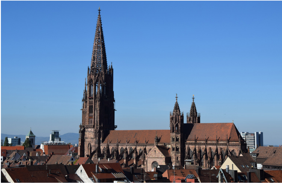
Fig. 1. Freiburger Münster, view from south, with its three openwork towers.
